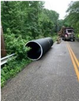
*The culvert that failed during Tropical storm Elsa was repaired within a week.*
