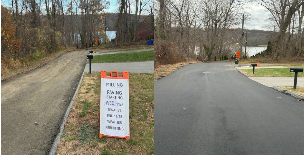
Standish Rd. after milling and after new paving
