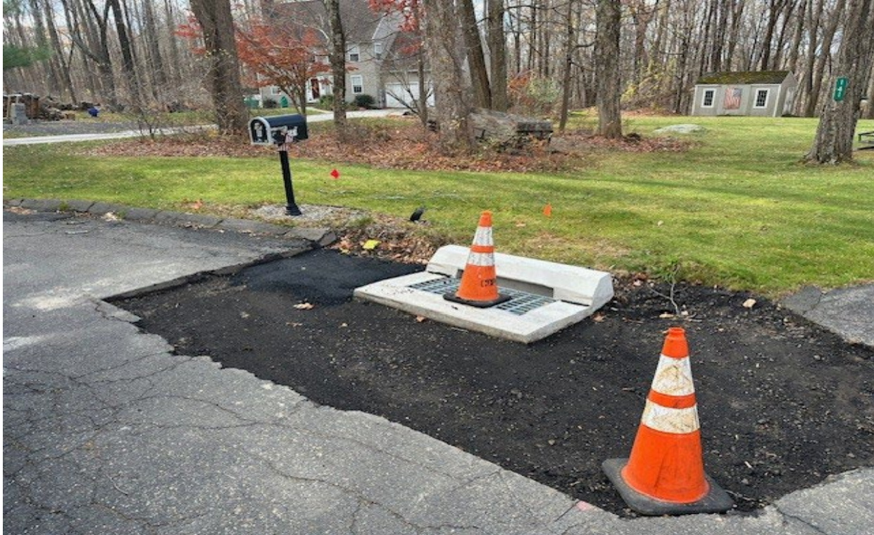
Leslie Lane drain replacement
