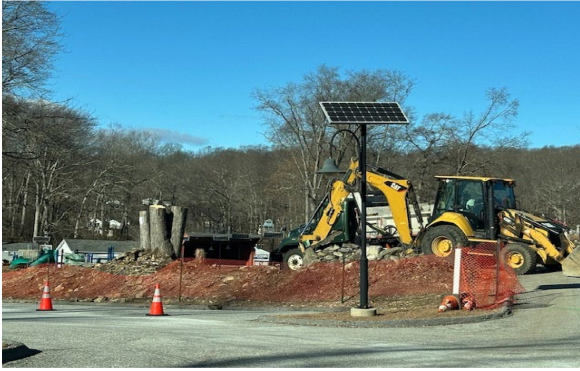
Patriots Park Playground earth work being done (adjacent to Senior Center/Lodge parking)
