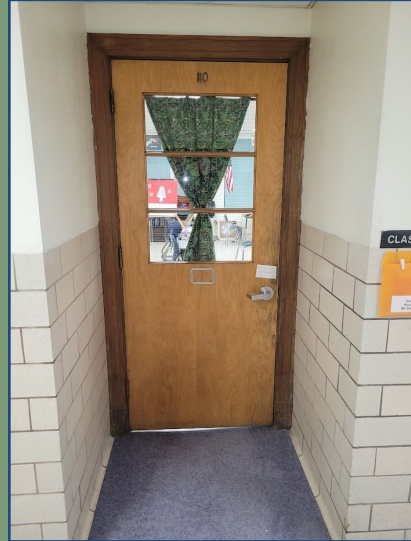
Original Classroom Doors 3rd & 4th Grade Wings 1949
