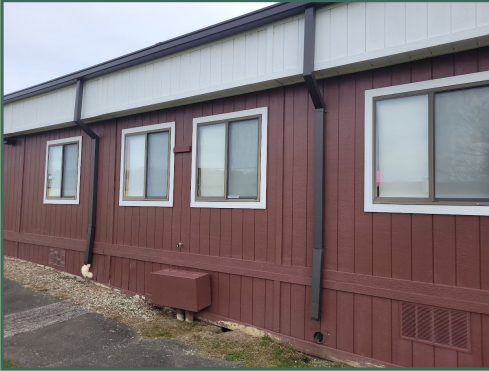
HEEC Original Siding - 1984
