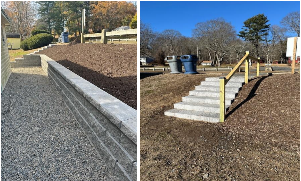
Lisicke Beach new wall and with completed steps with rail with solar lights
